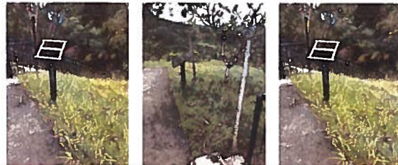
Overgrown greenery, mildew/algae on staircase, unutilized signage
