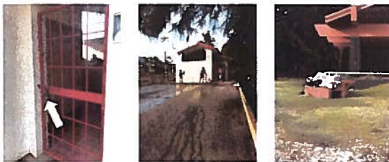
Inarajan Pool Inaccessible restrooms, neglected public showers, lack of garbage bins
