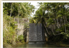
Fonte River serves as a natural border between the villages of Agana Heights Maaha. Prior to World War II in 1941, water from Fonte (also known as Libugon) Dam was the main fresh water source for Guam's capital. Photo by Victor Consaga/Guampedia
